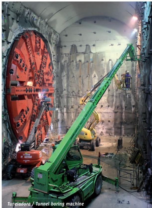
Tuneladora / Tunnel boring machine
